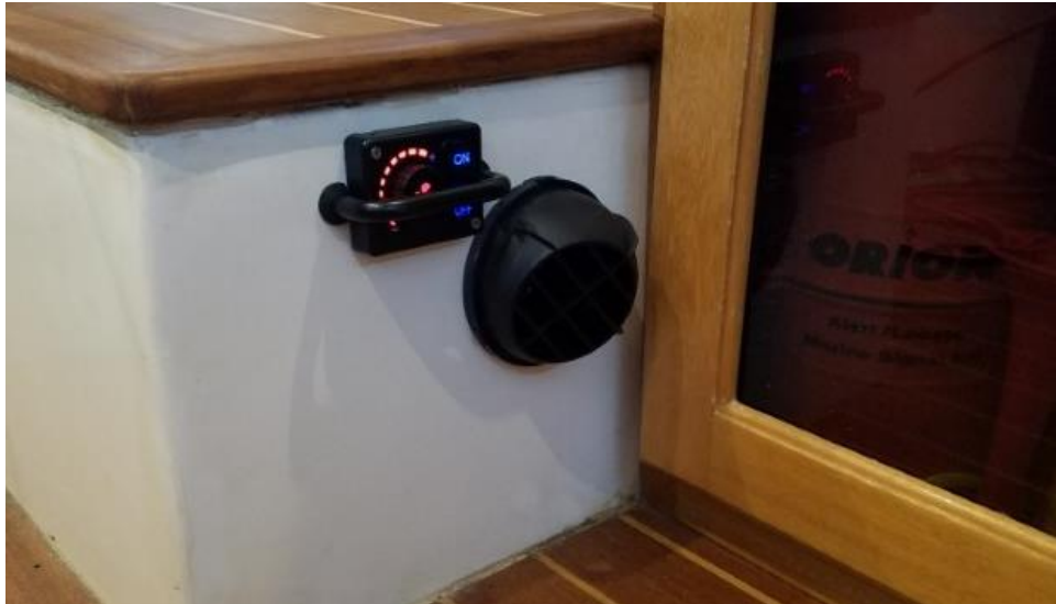
Hot Air Outlet Vent and Control Head
