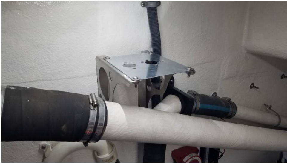
Shelf Brackets and Heater Base Plate
