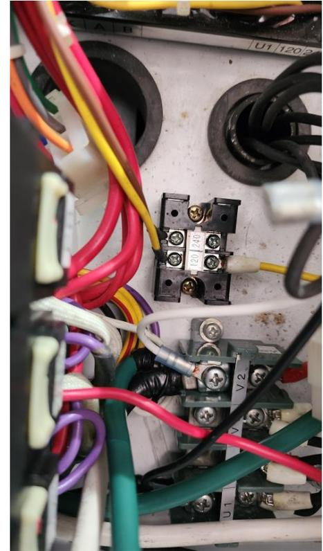
**Universal AVR. Note – generator was run approx. 3-hours under load using this AVR. Consistent out put of 125VAC/62hz per Blue Seas M2 monitor**
