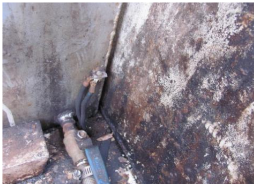
Steel and aluminum tanks likely in contact with each other
