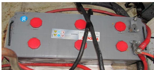
No box, no fuse, no terminal protection
