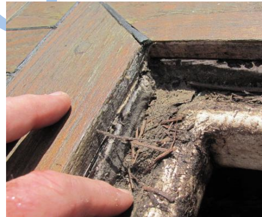
Deck hatch gutter without drains
