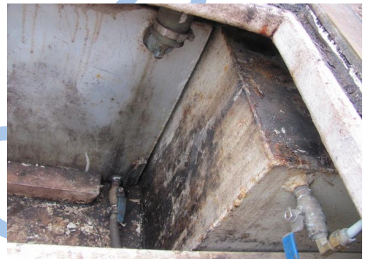
Steel and aluminum tanks likely in contact with each other
